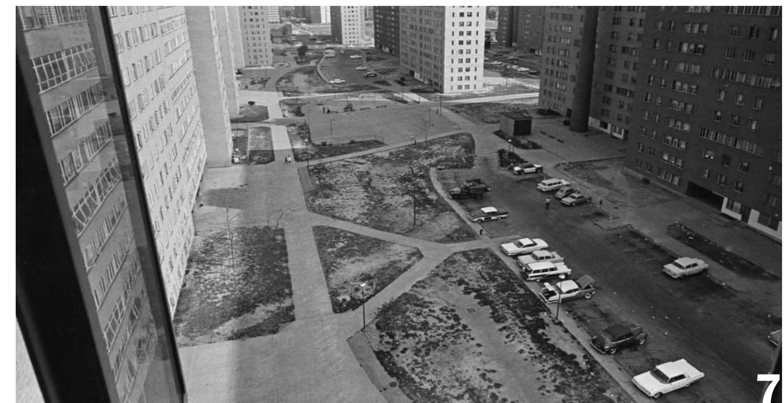
View of Pruitt-Igoe courtyards, Aug. 21, 1964. Photo Courtesy of PD&R Edge Magazine
