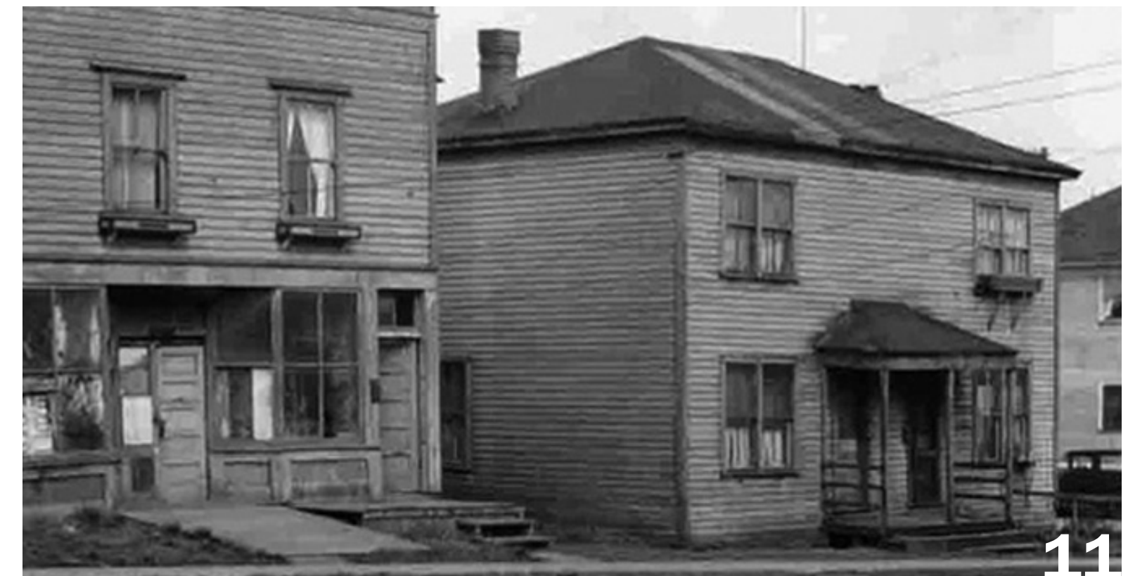
Close up view of Housing in Yessler Terrace (Photo Courtesy of Lawton Gowey)
