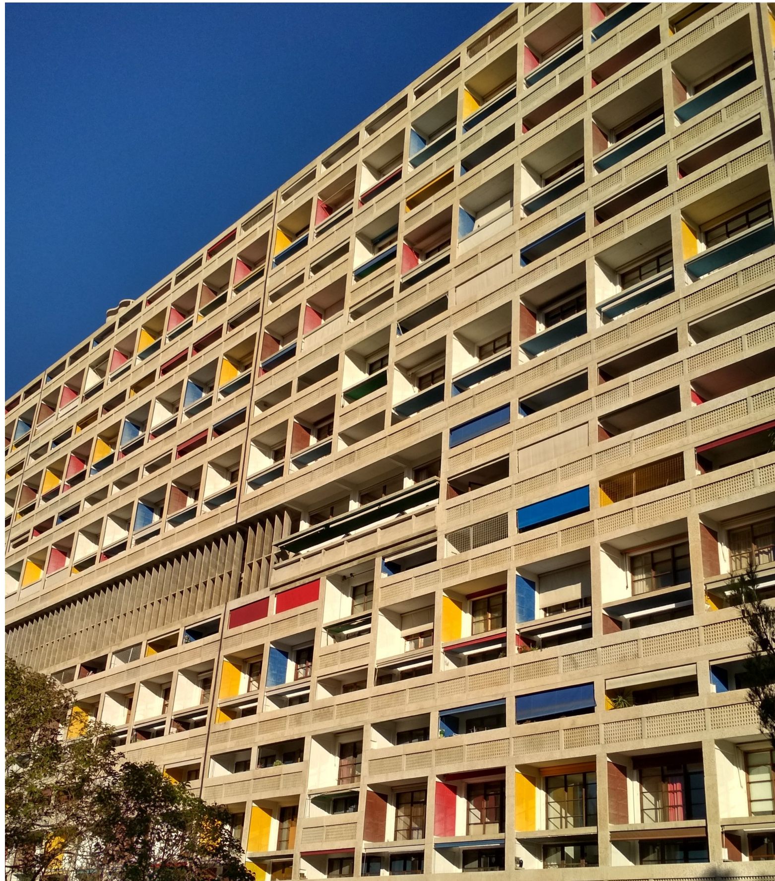
Facade of Unite d' Habitation by Le Corbusier (Photo Courtesy of Le Corbusier Foundation)
