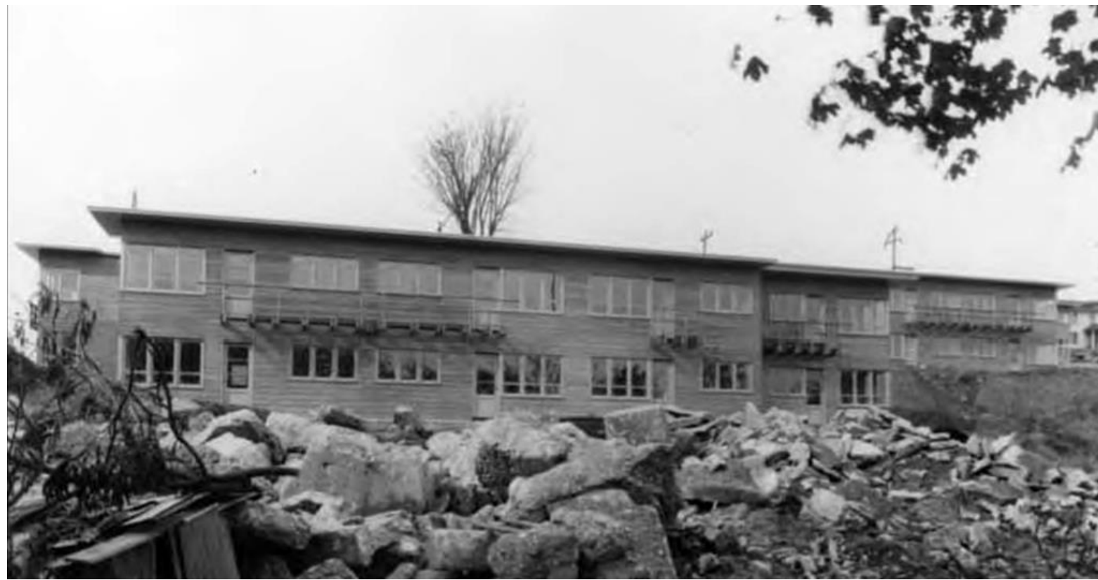
South facade of Yessler Terrace Housing (Photo Courtesy of Lawton Gowey)
