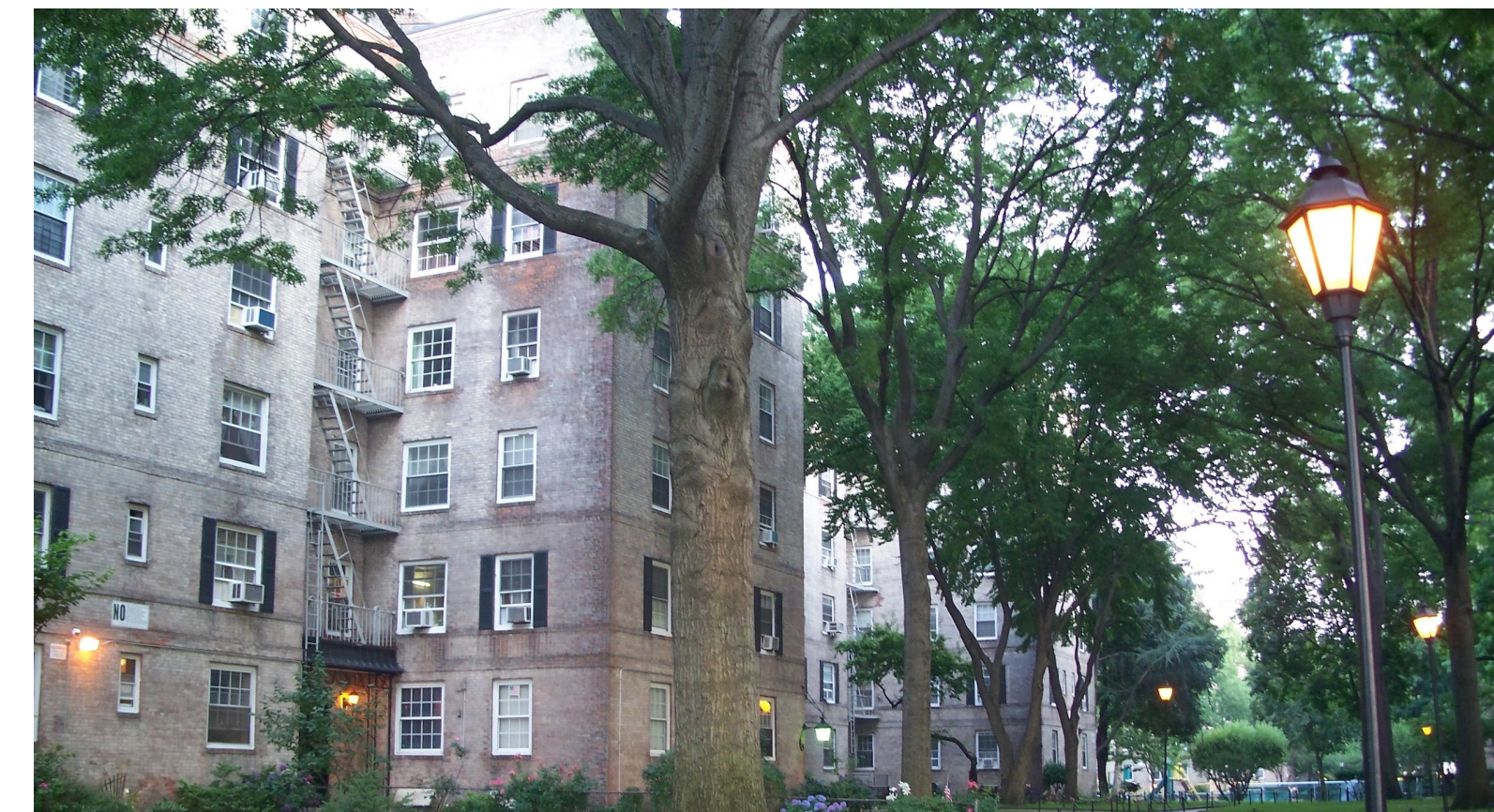
South Facade and Fire Stair of the Boulevard Gardens complex (Photo Courtesy of Apartments.com)
