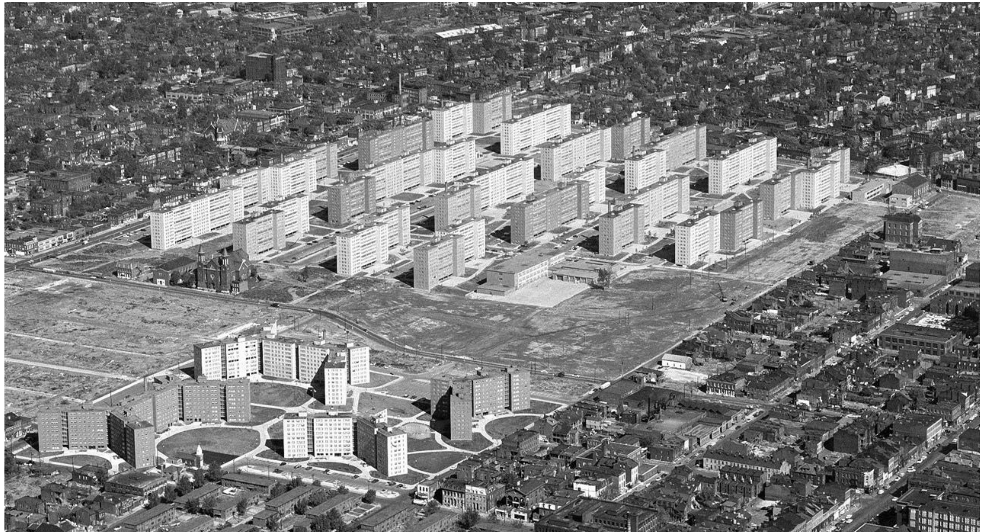
Aerial view of Pruitt-Igoe site, Oct. 11, 1964. Photo Courtesy of PD&R Edge Magazine
