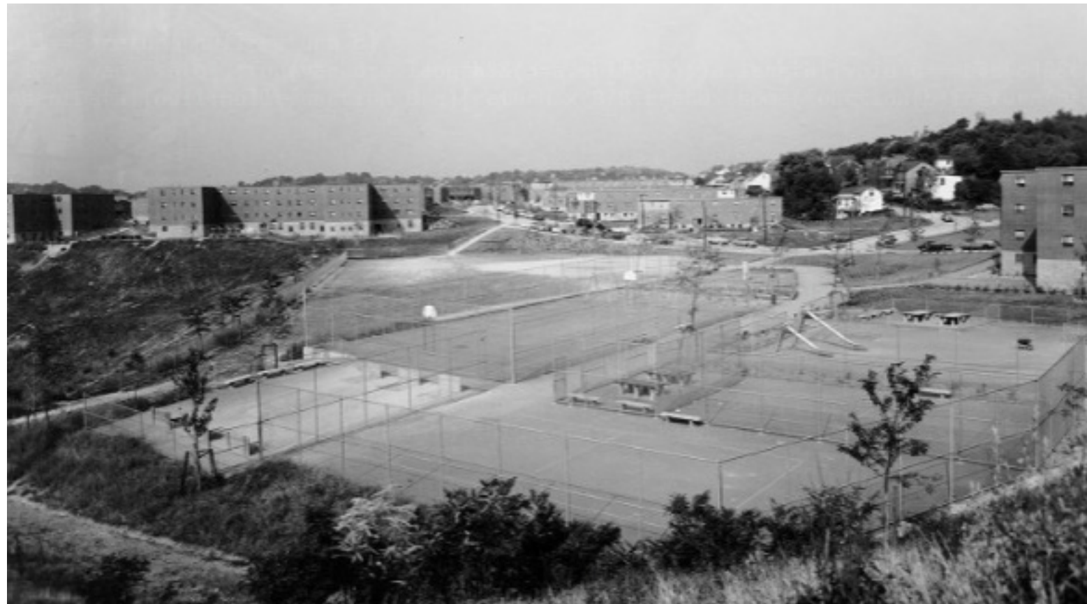
An aerial shot of St. Clair Village Parks in 1967. (Photo courtesy of the Allegheny Conference on Community Development Photographs, Deter Library & Archives, Heinz History Center)
